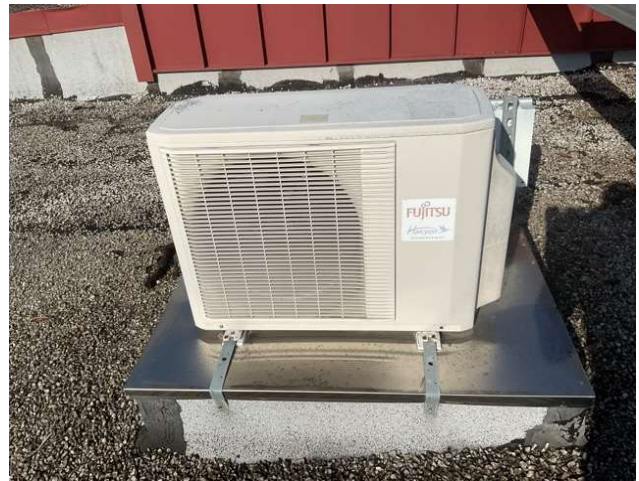
22 - SPLIT SYSTEM DUCTLESS
