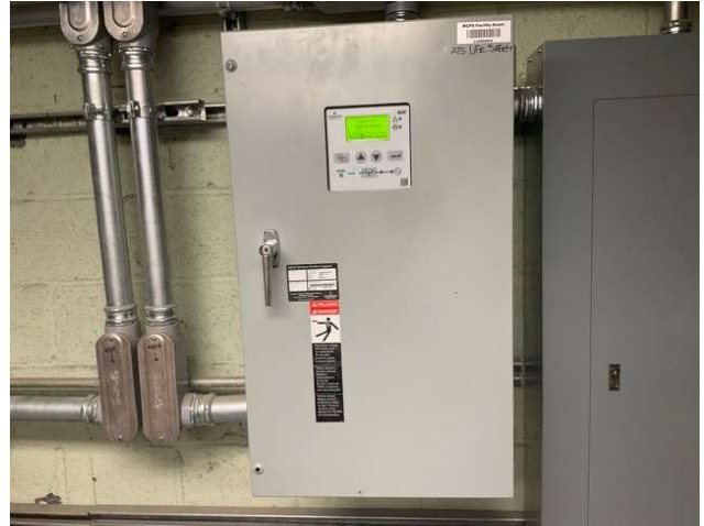
26 - AUTOMATIC TRANSFER SWITCH
